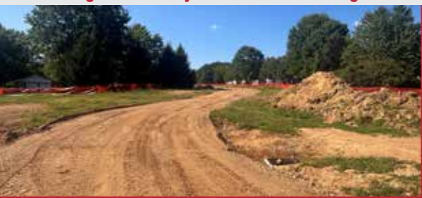
Rough grading on the new trail from the bridge through The Colony to The Keifer Building.
