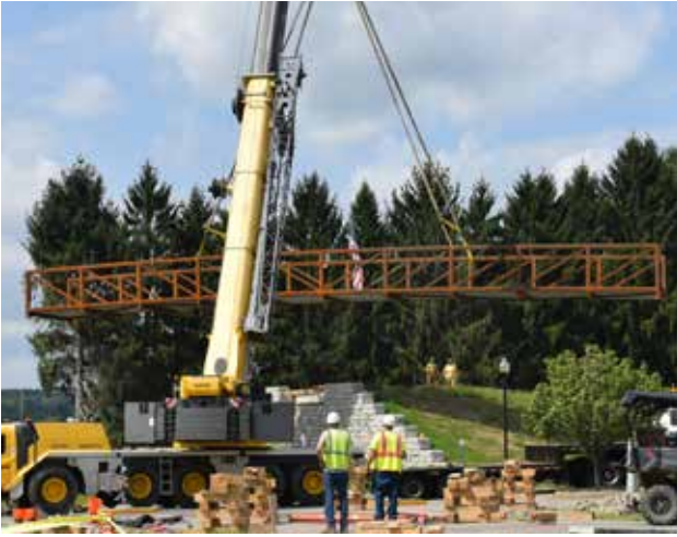
The bridge is raised into position.
