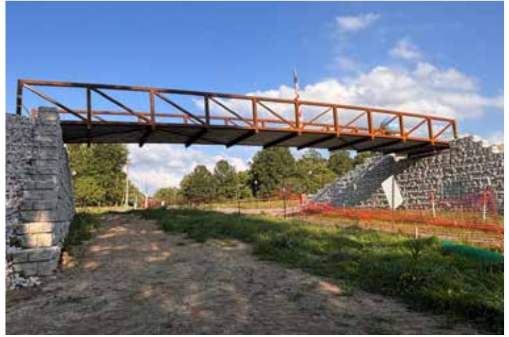
The bridge in place over Williamson Road.
