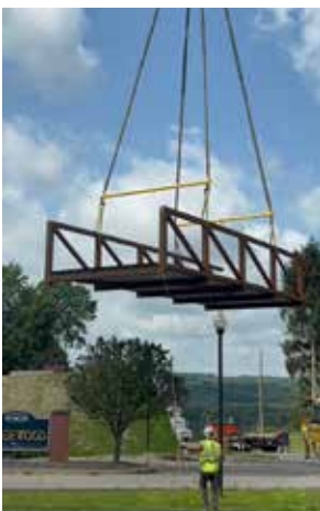
The second section of the bridge is lifted from the truck.
