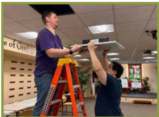
Paul Jewell & Erica Gulentz of our IT Department worked together to install the new ceiling speakers.
