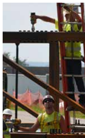
Crews get to work assembling the bridge.
