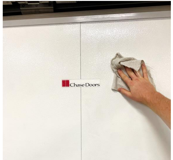
39. Clean door & track hood with wet rag.
