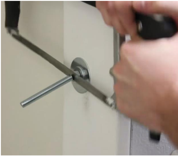
36. Cut off & file excess bolts.
