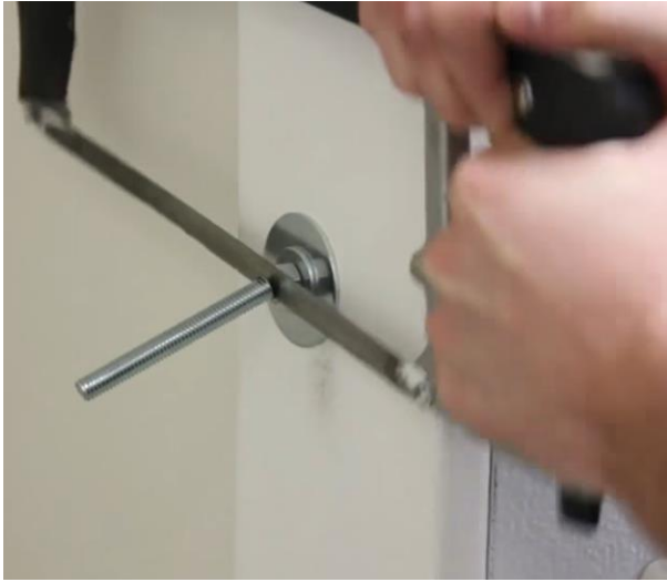
36. Cut off & file excess bolts.
