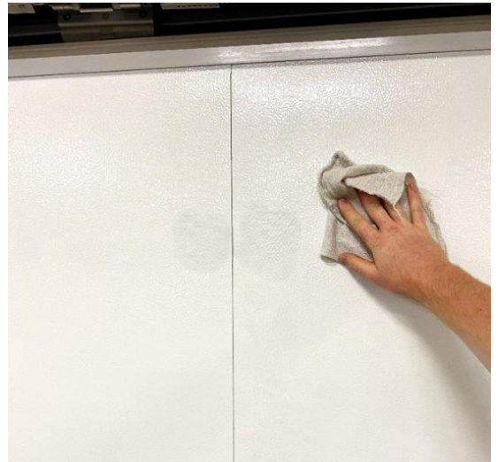
47. Clean door & track hood with wet rag.
