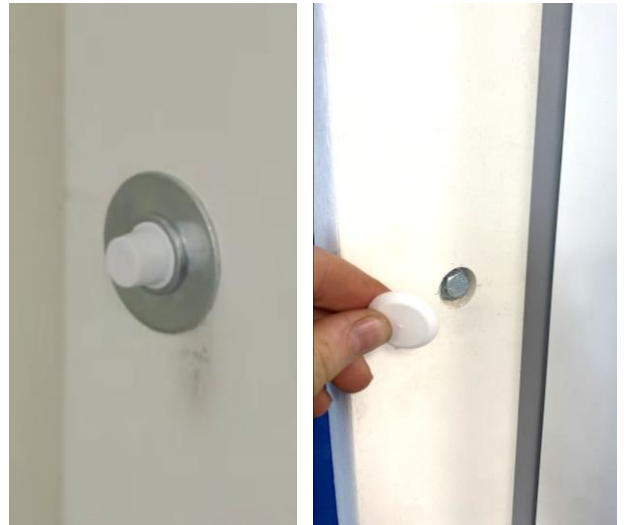
45. Install plastic white covers over the nuts on the inside and recessed holes on the outside face casing.
